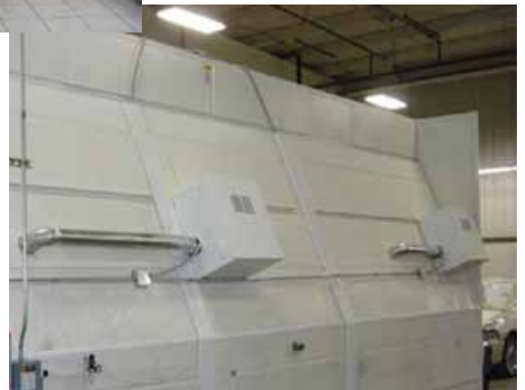
External view of horizontal retrofit tower remote motors
