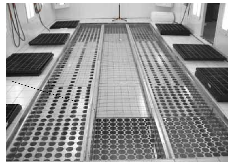
Optional 3-row exhaust pit shown here, grates and filters removed
